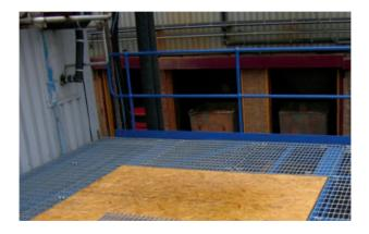
The notches made on the load-bearing sheet bars maximizes the nonslip. The sheet bars used in the distributing direction improves the strength of grating.
