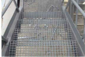
The round holes on the nosing ensures nonslip of feet. It is the most preferred type for strength. Optionally, it is hot dip galvanized, or painted, or manufactured without coating.
