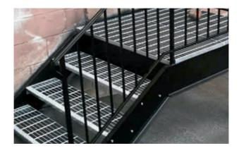
The steps contain extra mounting faces and nonslip nosing as compared to platform grating. The mounting face allows easy mounting of steps on the profile.
