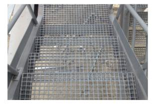
Double-sided notched full pass platform grating is typically chosen for environments where there is excessively slippery materials.
