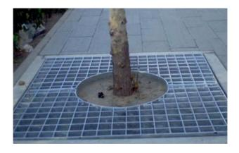
It is the most preferred type of platform grating for its appearance and strength. It may be manufactured in different dimensions of load-bearing and distributing sheet bars.
