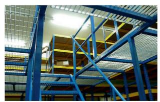
It is the most preferred type of platform grating for its appearance and strength. It may be manufactured in different dimensions of load-bearing and distributing sheet bars. Optionally, it is hot dip galvanized, or painted, or manufactured without coating.
