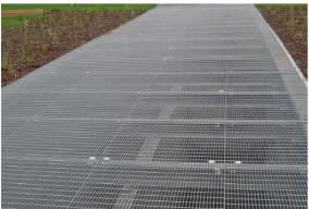
Optionally, it is hot dip galvanized, or painted, or manufactured without coating.
