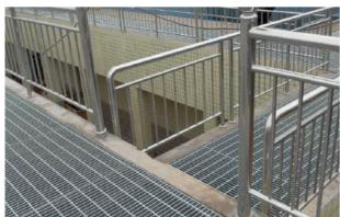
The round holes on the nosing ensures nonslip of feet. It is the most preferred type for strength. Optionally, it is hot dip galvanized, or painted, or manufactured without coating.
