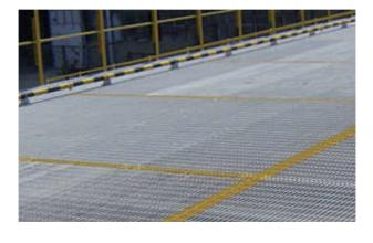
It is manufactured using transversal and longitudinal sheet bars of same size. It is heavier than the square twist and half pass platform grating.
